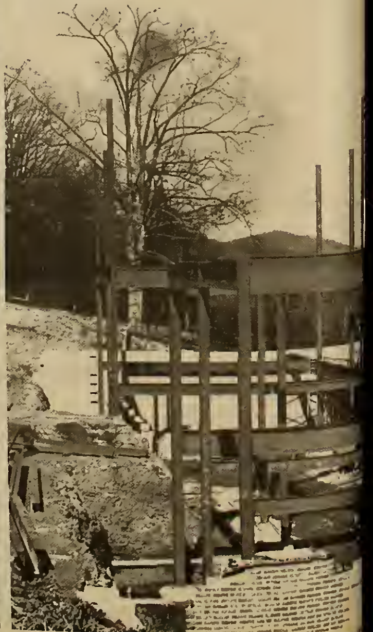
Steel frames of the new cafeteria building.
