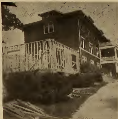
Jones Hall, with the southern wing still under construction.
