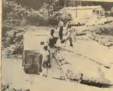
The Bridge near Antillian College in Puerto Rico was destroyed last year in a flood. Photo by Gary Moore
