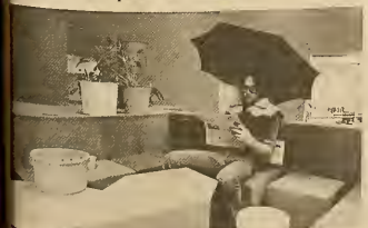
The atmosphere of the outdoors is liberally brought indoors in the Student Center. Due to a leaky roof, flash flood are not uncommon.
