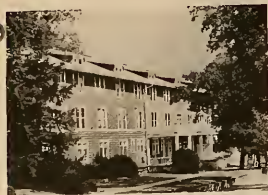
Maude Jones Hall, first occupied in 1917, was razed last week. After the English Department departed to Brock Hall during the Christmas vacation, the building had
