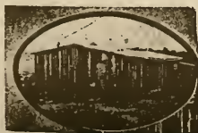
A temporary structure used by the boys. They often work until midnight standing under and above lights in order to abbreviate as much as possible their minutes in each quarter. Many would not think of spending any time in such buildings.
