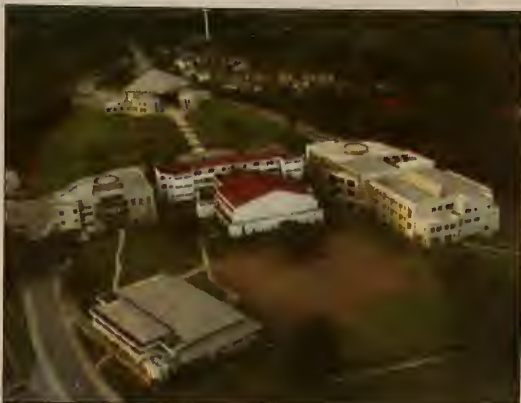
This is an aerial view of the Mission College campus.
