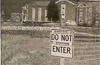
This shot overlooks Talge East where the new wing will be added. Fifty parking spaces were lost when the lot that used to be here was destroyed to make room for the new wing.
