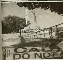
Construction at Talge dormitory Photo by Kimberly Stabel
