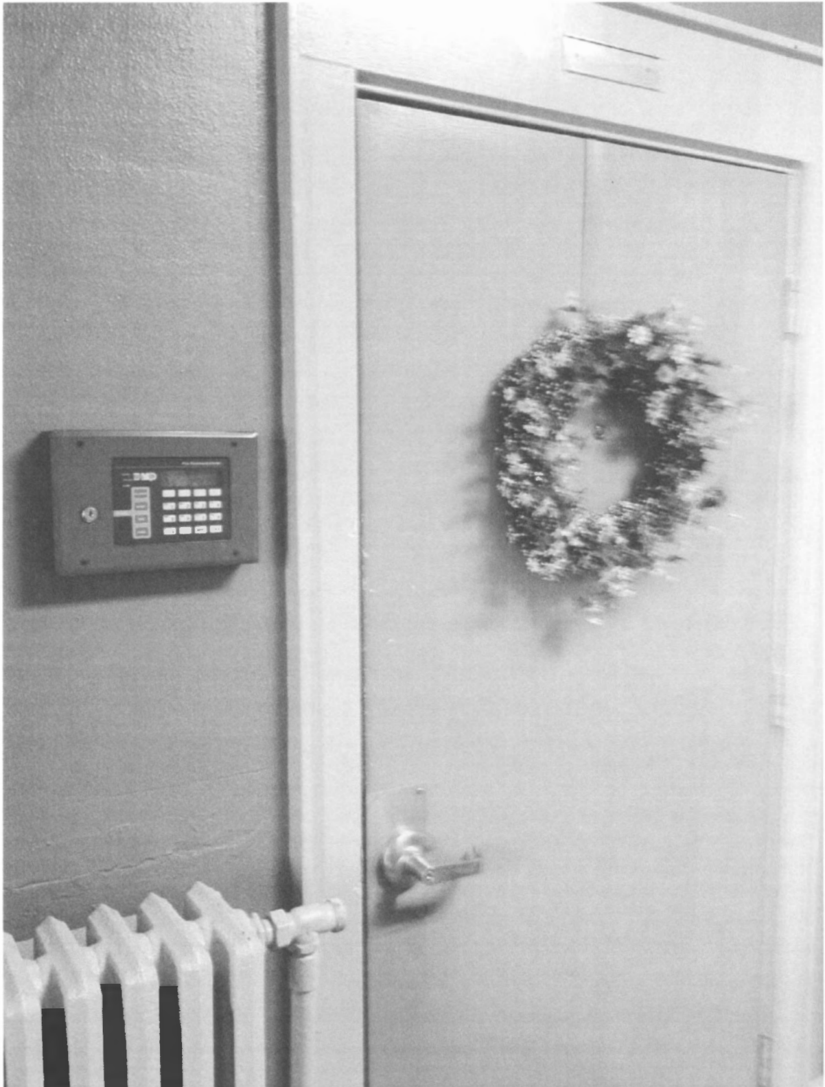
Insert Electrical Room Map-Suite 12 inside Main Entrance
