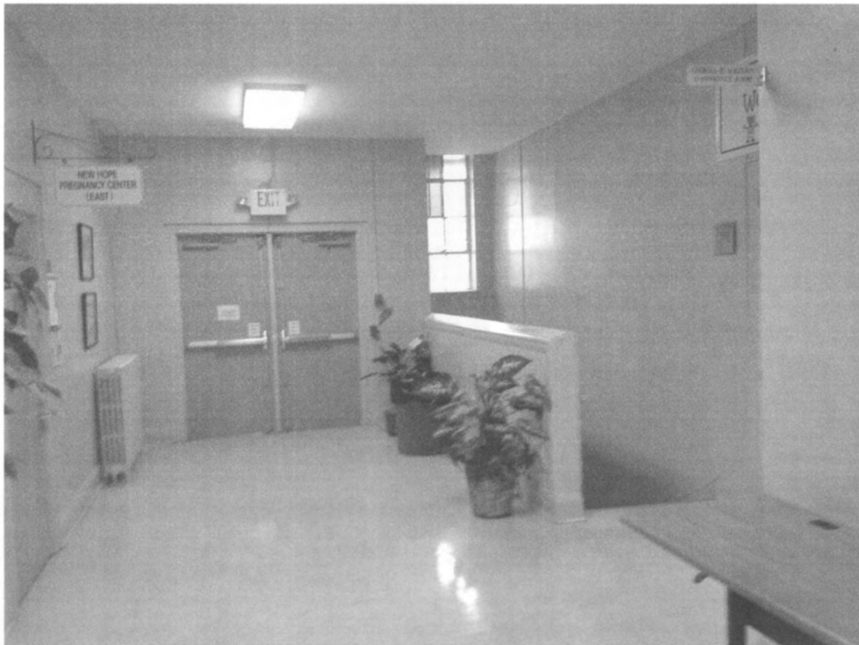
Fire Extinguisher Outside NHPCC – behind plant
