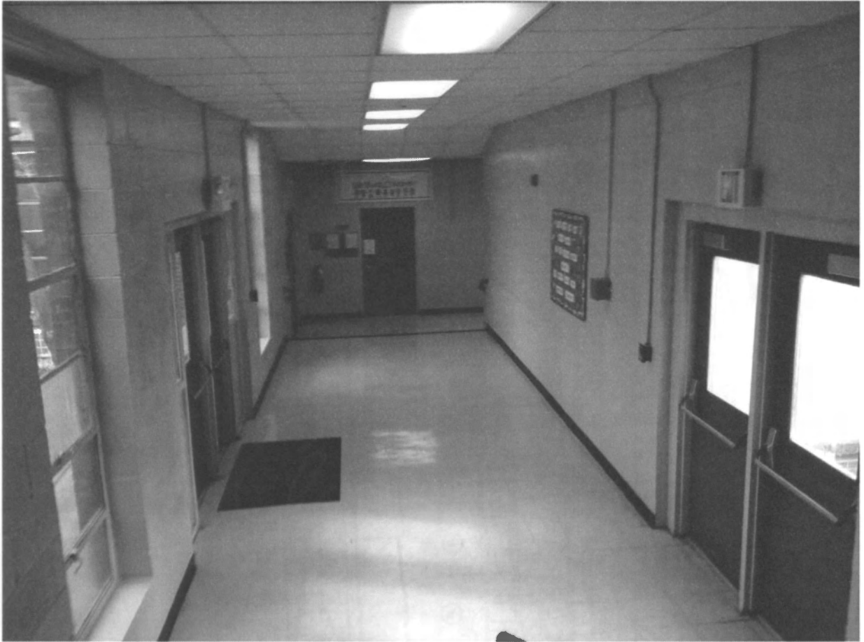
Fire Extinguisher @ East End through double doors
