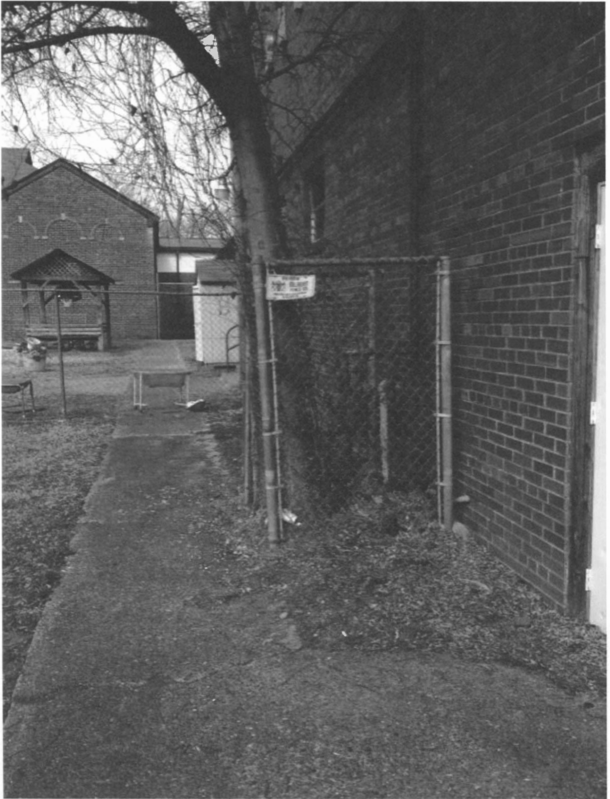
South Side of Building
