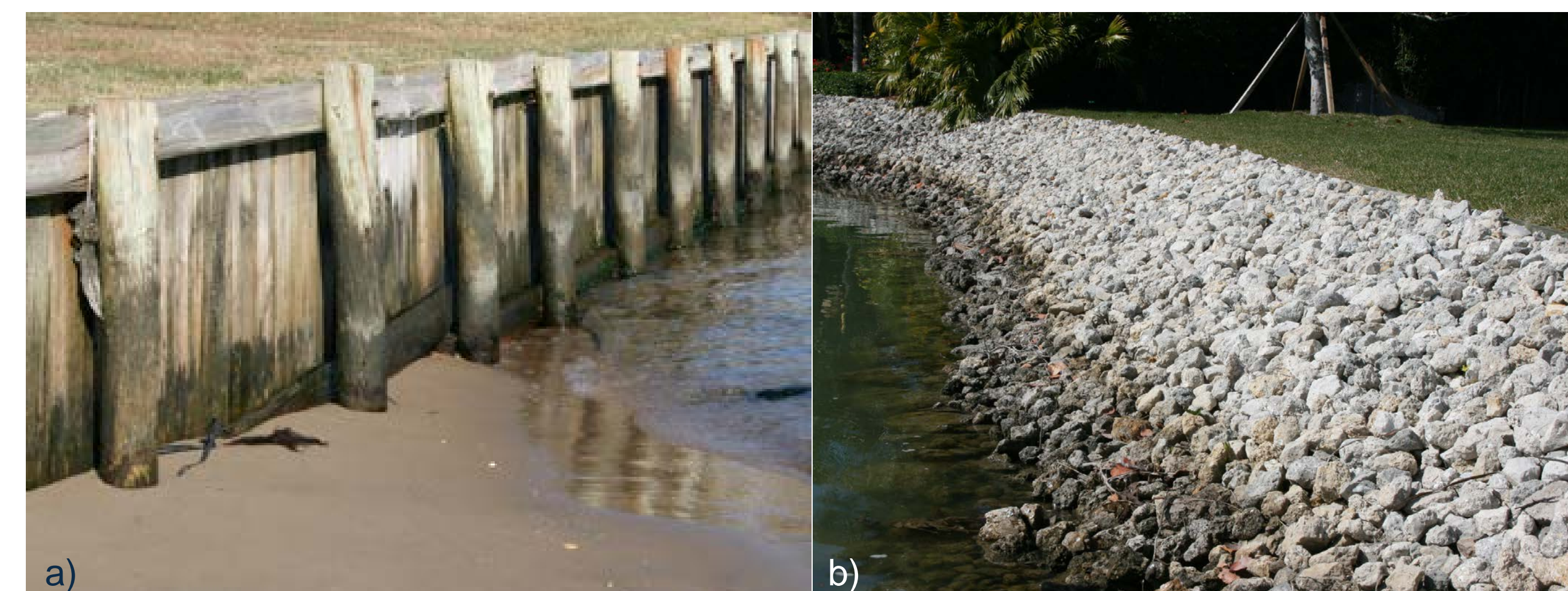
Figure 1: Bulkheads (a) and riprap (b) are common methods of shoreline hardening. Both methods stabilize shoreline erosion, but also limit inland migration and accretion of wetlands. Source: VIMS.
