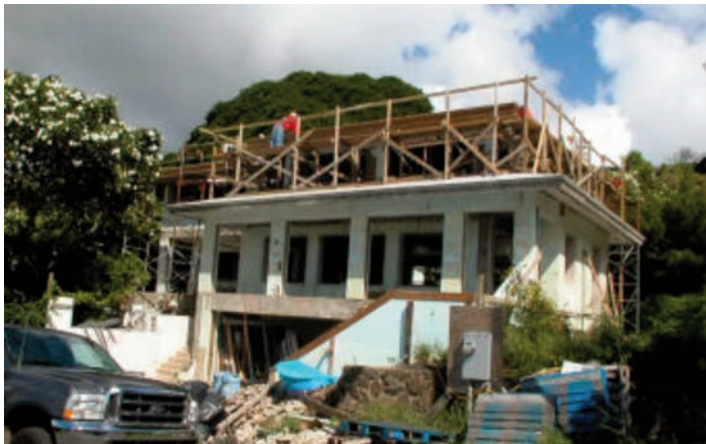
A residential home being constructed in Makiki
