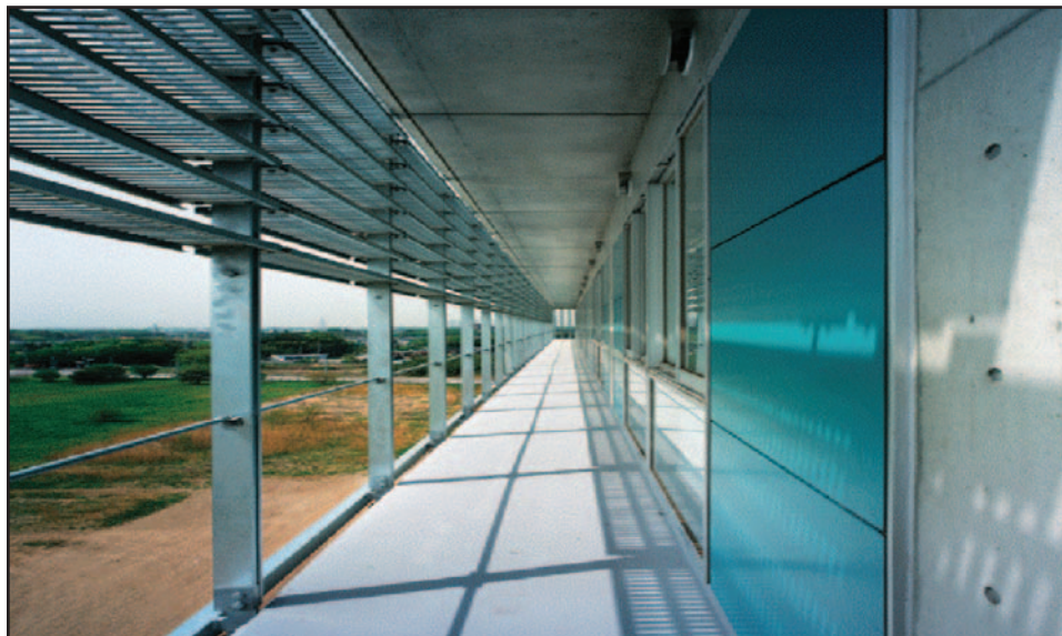
Figure 3 Building Envelope showing shading and ventilation for energy savings, Kashiwa Campus, University of Tokyo
