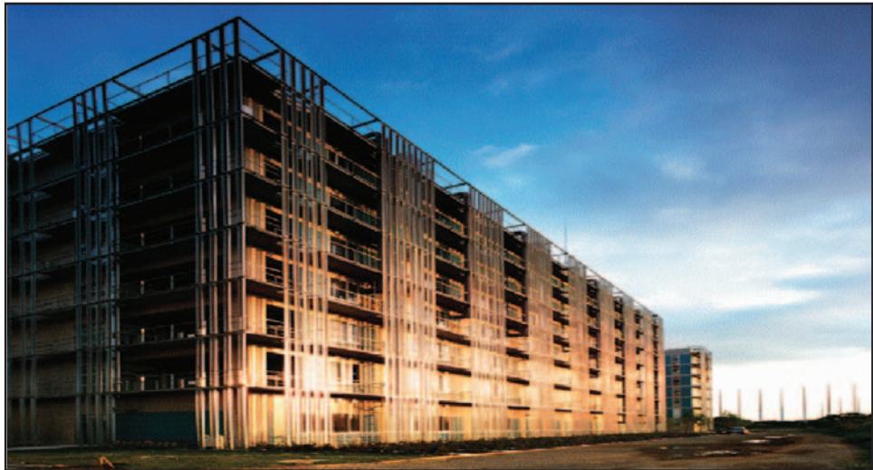
Figure 4 Building envelope showing the louver design for energy savings – Kashiwa Campus, University of Tokyo
