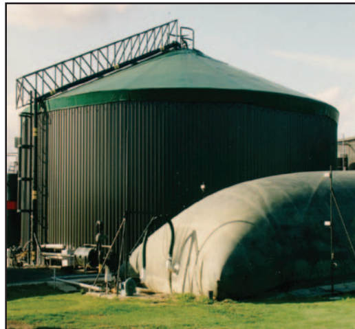
Figure 1 Methane capture at a Brazilian landfill
