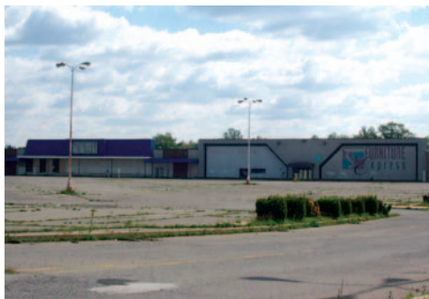
Willingboro – Empty Strip
