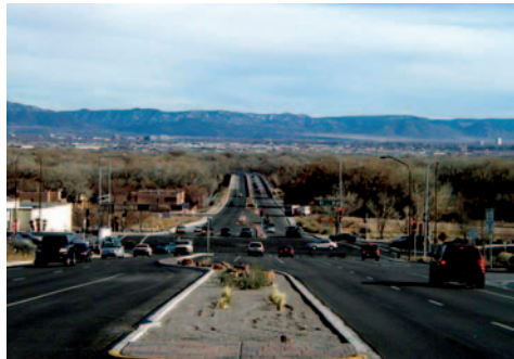
Montano Bridge, Albuquerque
