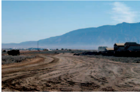
Road Construction to Sprawl
