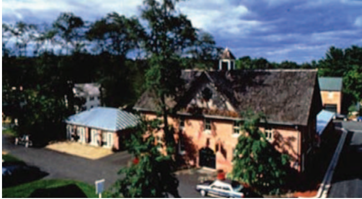
An aerial view of the Old Farm Neighborhood Photo courtesy of Duany Plater-Zyberk
