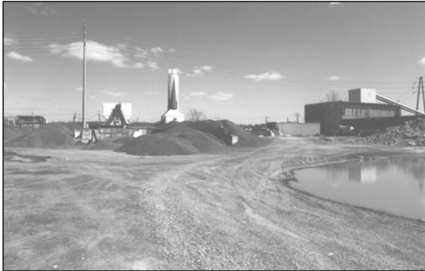
Figure 9 L. Suzio Concrete Company
