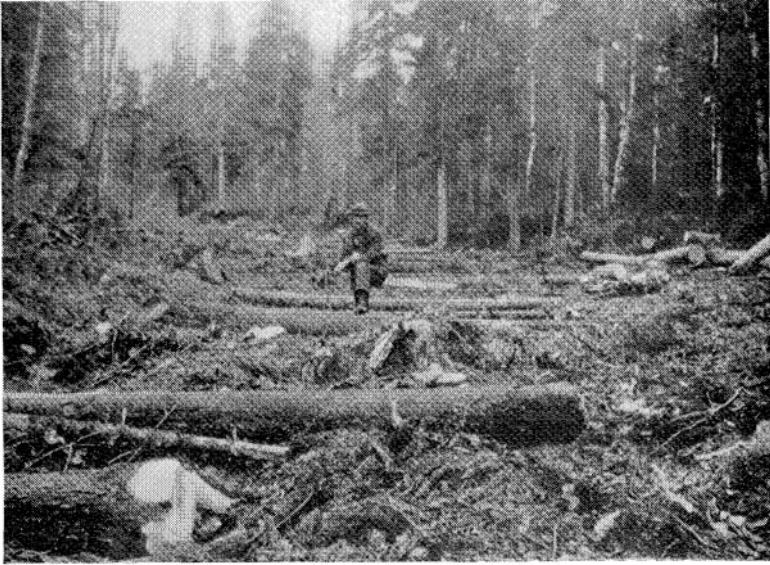
Fig. 11. The Roadbed for an Iced Road which is to be built upon a Deep Snow Foundation.
