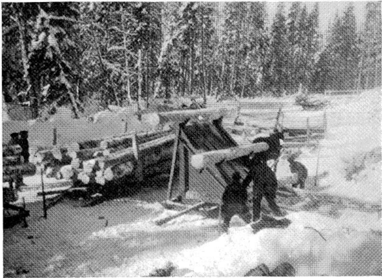
Fig. 45. A Power Conveyor driven by a Gasoline Motor used for loading Logs on Sleds. Eastern Canada.
