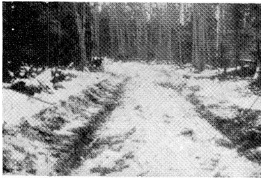
Fig. 22. The appearance of a Rut Road before it has been used for the first tilne. The ruts have been cut in the earth follo\ving a light snowfall. I\linnesota.
