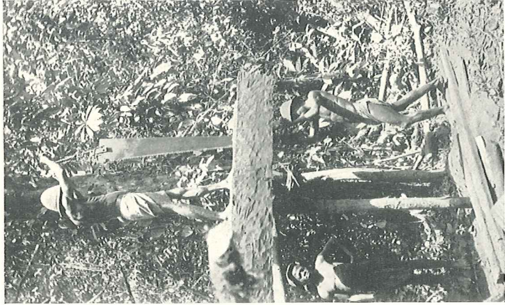
Plate XIV. No. 1. Pit-sawing hewed logs into planks.
