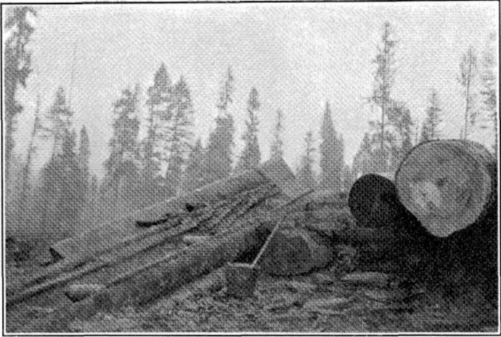
Fig. 20. The intake of a V-chute equipped with dead rollers.
