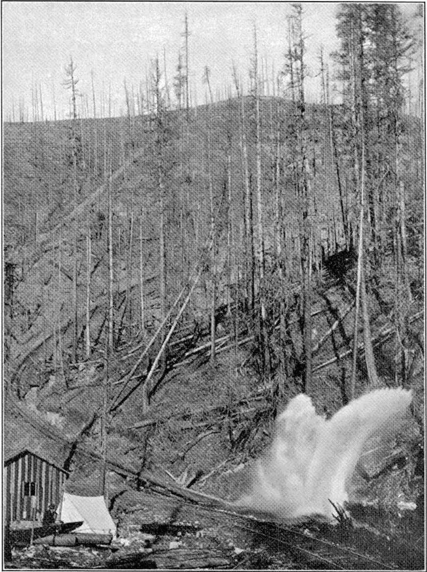
Saw logs moving down a V-chute and discharging into a pond along the logging rail-road. St. Joe National Forest) Idaho. (Photo by courtesy U.S. Forest Service.)
