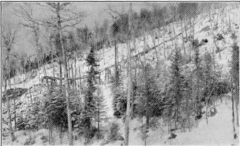
Fig. 9. A typical pulpwood pole chute discharging wood from a trough elevated on a trestle bent. Eastern Canada.
