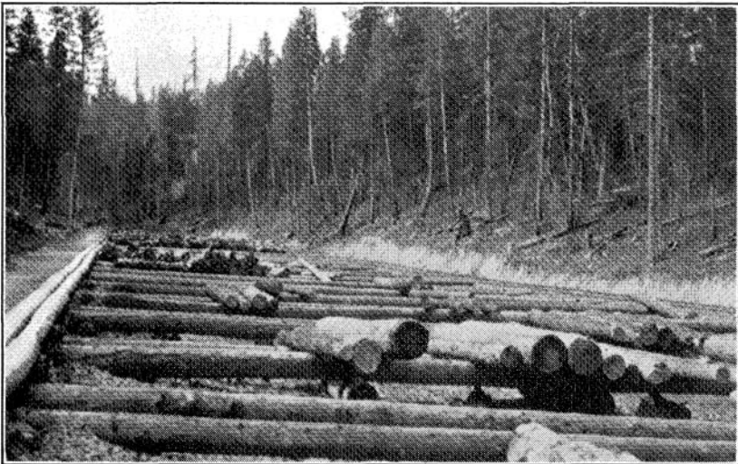
Fig. 21. A trailing chute landing along a logging railroad. Montana.
