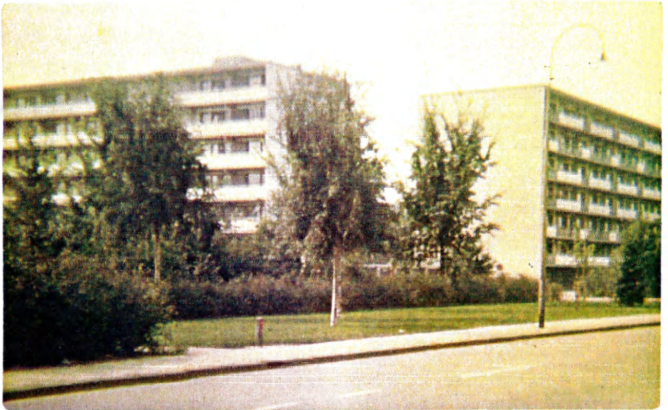
Illustration #2: The Flats - modern apartment complex.
