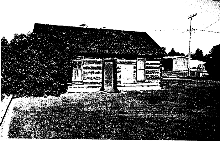
Figure 7:7 Greenwood Ranch Station Building (Dalton Museum)
