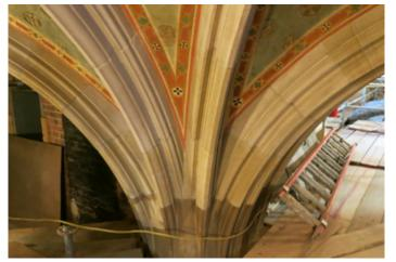
Detail of a stone arch at the nave ceiling; stone that has been cleaned forms a stark contrast with stone that has not. **Photo by Amanda Patrick**
