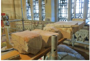
Examples of some of the deteriorated stones from the walls of the nave; after damaged stones were removed, they were replaced with carefully crafted replicas. **Photo by Amanda Patrick**
