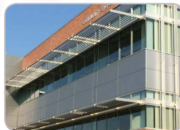
Figure 34: The Community Engagement Center was designed to provide plenty of access to daylight, and its awnings and shades allow for the sunlight to be appropriately managed. The CPACS building does not have awnings, but its occupants can (but sometimes don't) use shades to manage the sunlight.
