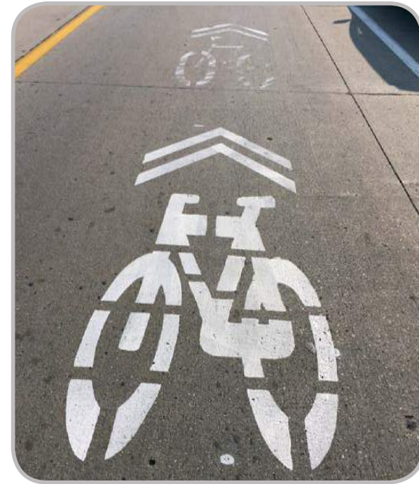
Figure 28 Pacific Campus already has “sharrows,” but bike routes on Dodge Campus currently lack them.
