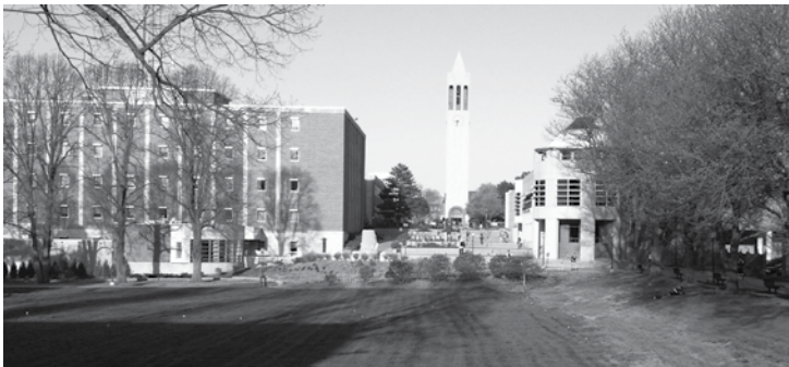
Existing Conditions of the Pep Bowl looking west
