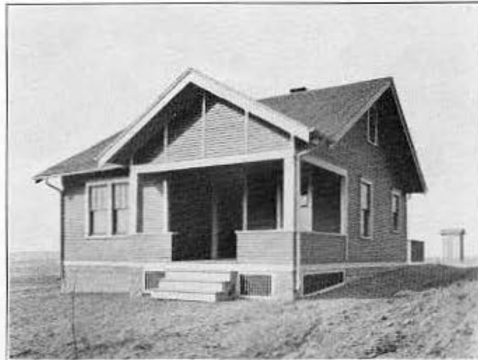
No. 266 —This Cottage is built in Benson Gardens, which is located one mile west of the city of Benson. It has four rooms and bath, same making an ideal home for city farmers. This house can be built for about $1,600 00.
