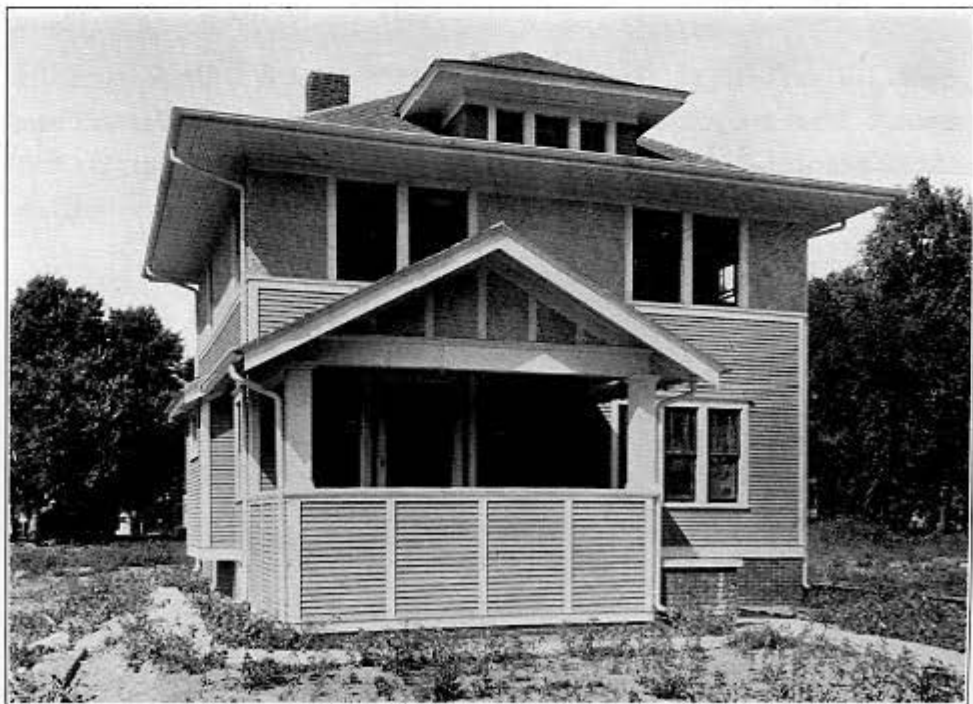
No. 235 —For a Moderate Priced House this is a very good example. With its hip roof, wide cornice and gable porch it is very attractive. There are six rooms and bath in this house and the building is 24x26 feet, outside measurements, with a 10-foot porch. Can be built for $2,800.
