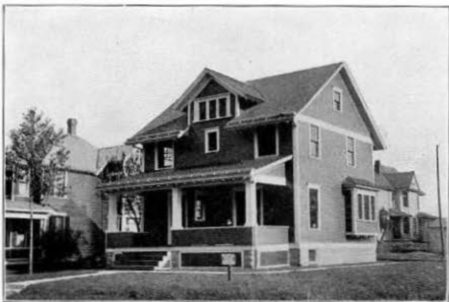
No. 239—For an Investment, a plain substantially built house is always very desirable. Large windows, large front porch and seat in dining room adds greatly to the appearance of the house.
