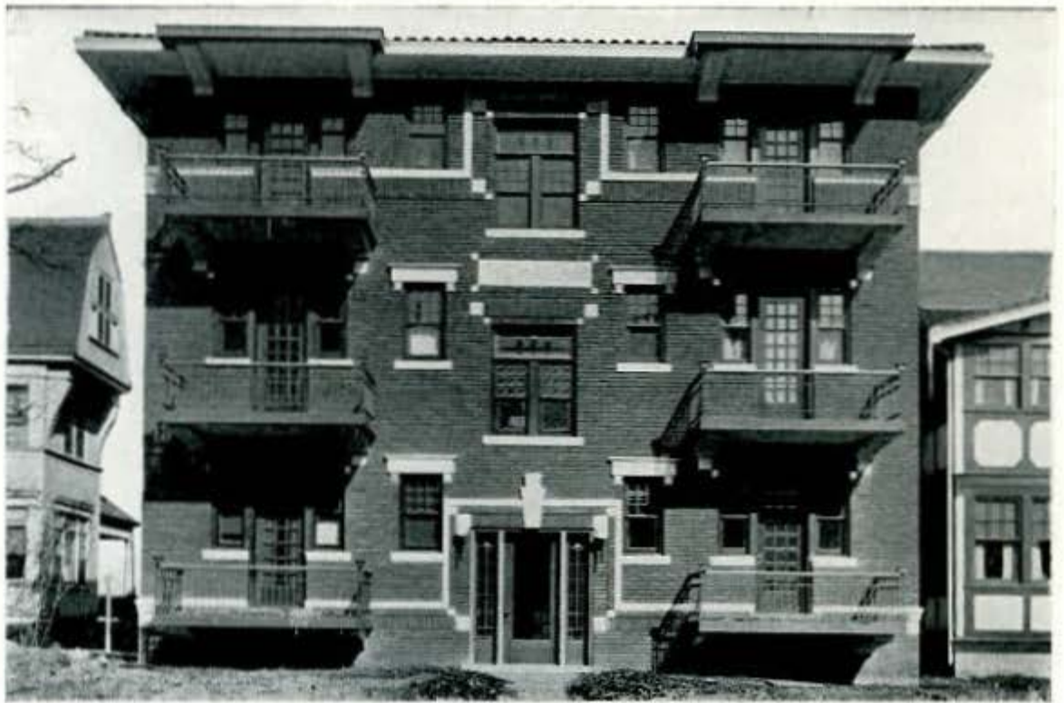
No. 209—Mayfair Apartments , located on Jackson Street, between Twenty-second and Twenty-third Streets. Owned by B. G. Bilz. Has twelve 3-room apartments, each apartment having private balconies. (Twenty-six Murphy In-A-Door beds used. National Roofing Company furnished tile and gravel roof. Milton Rogers furnished hardware. American Gypsum block partitions and American Plaster Board lath. American Electric Company furnished fixtures and wiring. Monarch weather strips used for windows. Building faced with Sunderland's Brazil X press brick.)
