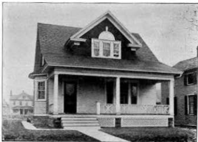
No. 240—This Type of House is very popular and has a character of its own. Main roof sloping over porch gives the house a squatty appearance and still leaves ample space for bed rooms on second floor.
