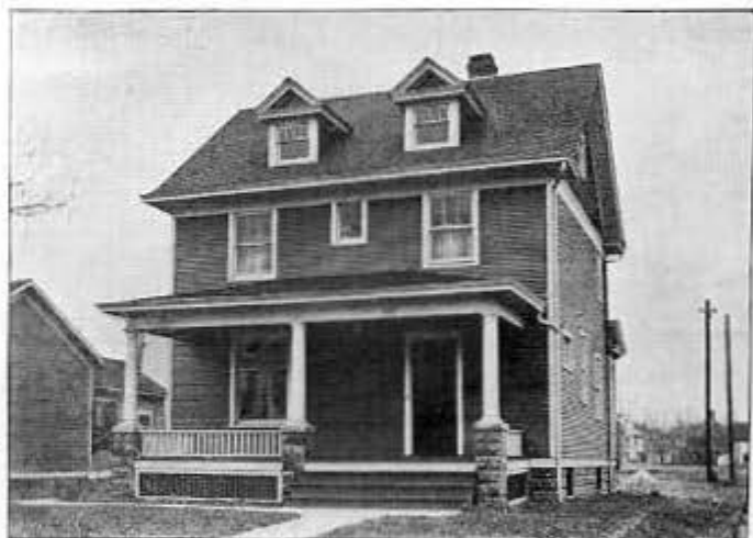
No. 246 —This Design is similar to No. 239, but this house can be built for considerable less money and still is an attractive looking house. All our house designs have built-in China cases, pantries, closets and other modern conveniences.
