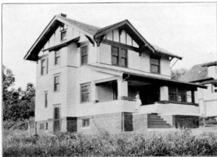
No. 241—This Beautiful House is 26x24 in size, has 7 rooms and sun-room, and designed for a moderate priced lot. Is built of frame with a press brick foundation.
