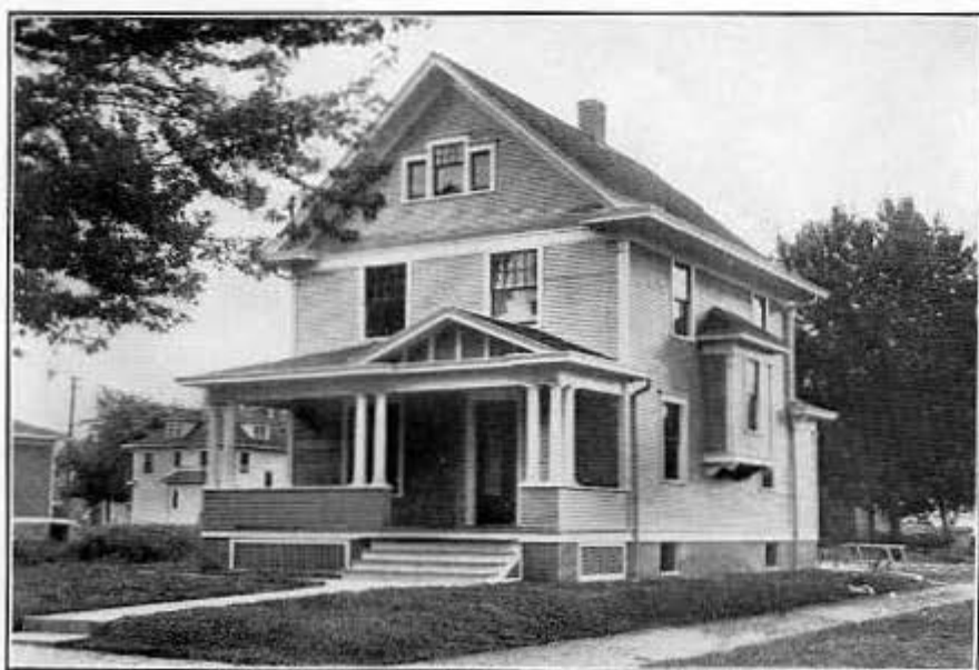
No. 247 —This Gable-roof House is inexpensive to build and also gives plenty of attic room with windows at each end. It has six rooms and can be built for $3,500.
