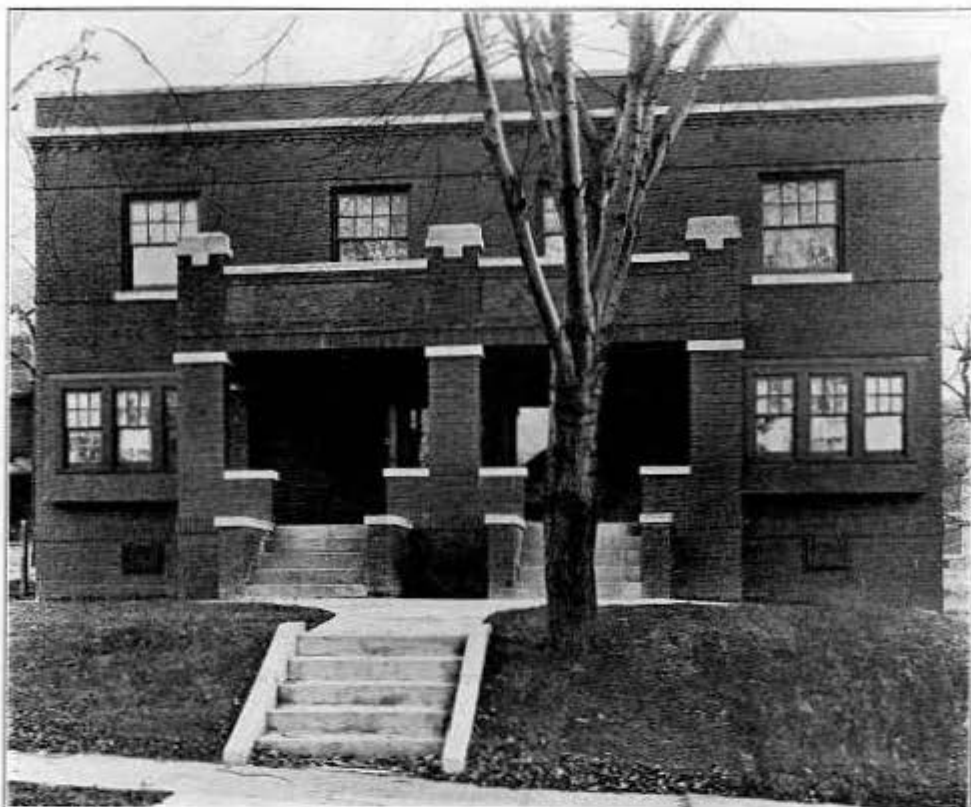
No. 232—A Double Brick Apartment like this has very little up-keep and is a safe investment. The apartment is owned by Mr. Roach and is located at Eighth and Williams Streets, and cost $6,500. Each apartment has five rooms and bath. Furnace heat.
