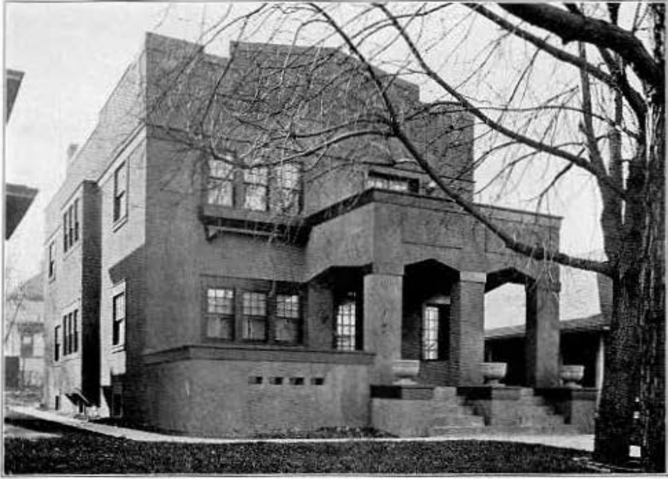
No. 226 —This St. Louis Stucco Flat was built for G. A. Greenough at Ninth and Williams Streets. It has two apartments of five rooms each and cost $6,000. This is a very good type of apartment for a narrow inside lot.
