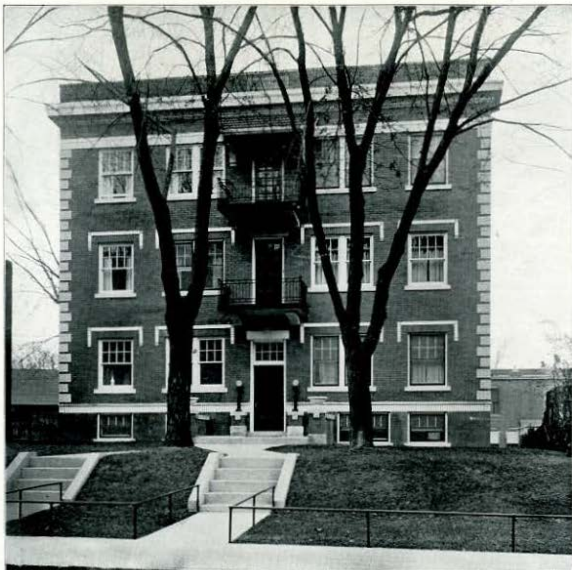
No. 208—Leigh Apartments , located on Twenty-fifth Avenue, between Farnam and Douglas Streets. Has twelve 4-room apartments. Is owned by Sam Mort. (American Electric Company furnished fixtures and wiring. Twelve Murphy In-A-Door beds used. Building faced with Hytex No. 550 dark press brick. Glauber brass ware used.)
