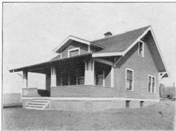
No. 267 —This Cottage is planned similar to No. 266. It is also built in Benson Gardens, but would make an ideal home for a moderate priced lot in the city.
