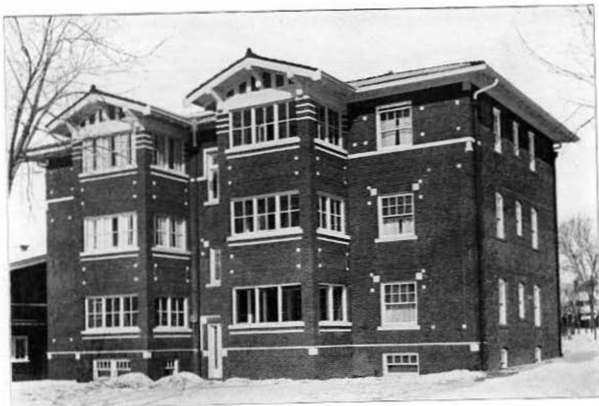
No. 217—Leeton Apartments , located at Forty-ninth and Dodge Streets. Has six 5-room apartments, each apartment having large private sun-room. Faced with Hytex No. 900 press brick.
