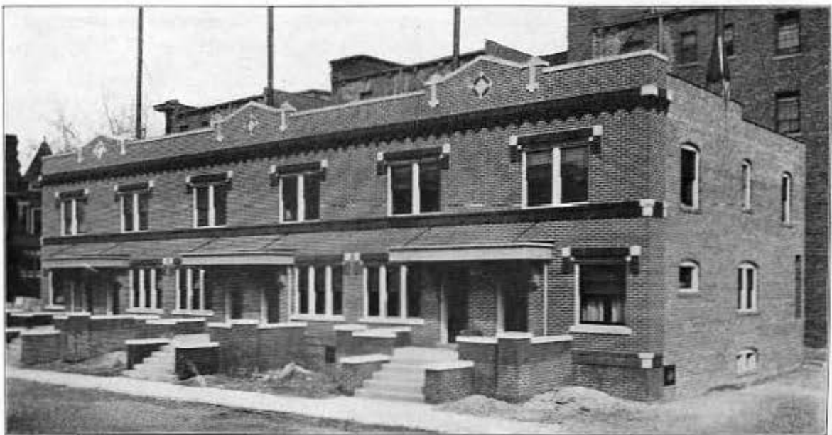
No. 220 —Paxton Court Terraces No. 2, located at the east side of Paxton Court and contains six 5-room apartments. Building erected and owned by Hastings & Heyden. (Glauber brass ware used. Murphy In-A-Door beds used. American Electric Company furnished fixtures. Faced with Hytex No. 430 face brick.)
