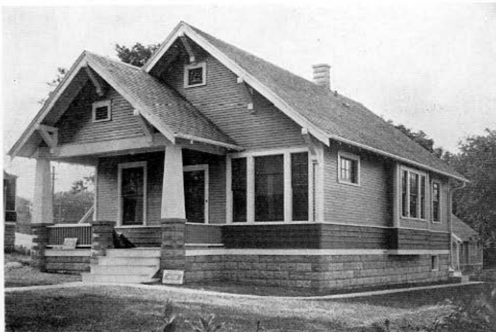
No. 258 —An Attractive and Inexpensive Bungalow with gable end porch; heavy brackets; cement block foundation. Has five rooms and can be erected for $2,200.
