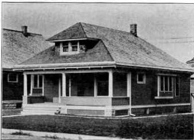
No. 261—This is a Very Good Illustration of a hip-roof, five-room cottage with main roof extending over front porch. The large dormers in attic give ample room for finishing off one good-sized bed room.
