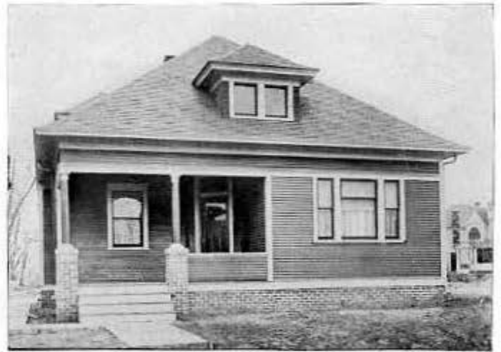
No. 260—Acreage Property demands four-room, inexpensive cottage of which this is a very good example. It is 24x30 and can be erected for $1,800. Has brick foundation and finished in Yellow Pine.
