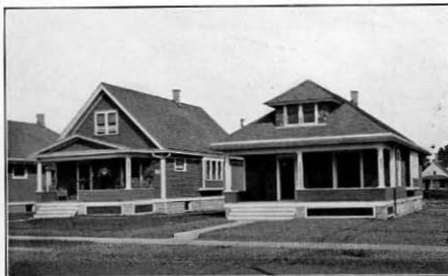
No. 264—These Two Cottages are suitable for moderate priced lots, or suburban property. They are very sensible in appearance, each having five rooms, large front porch and full basement.
