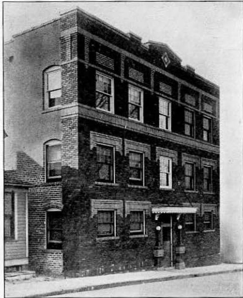
No. 221—Wayne Apartments , located on Dewey Avenue, east of Twenty-eighth Street, containing eighteen apartments of 3 rooms each. (Thew & Lahr installed electric wiring. Omaha Structural Steel Works furnished iron. Eighteen Murphy In-A-Door beds. Burgess-Grandon Company furnished electric fixtures. Faced with Hytex press brick.)
