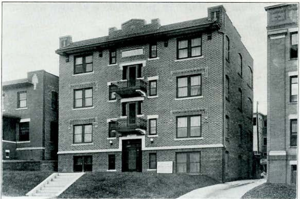
No. 205—Harney Apartments , located on Harney Street between Twenty-ninth Avenue and Thirtieth Street. Built and owned by Hastings & Heyden. Has six 4-room apartments and two 2-room apartments. (Thomas Rich, plumbing contractor. Eight Murphy In-A-Door beds used. American Electric Company furnished fixtures. Milton Rogers furnished refrigerators. Monarch weather stripping used. Faced with Sunderland's Brazil X face brick.)
