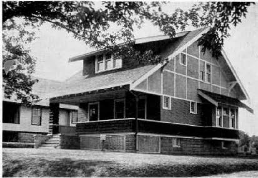
No. 265 —This is Another Type of House where main roof extends over front porch. The ends of gables are stucco wood-panel, which gives a very pleasing effect. Has six rooms and bath.
