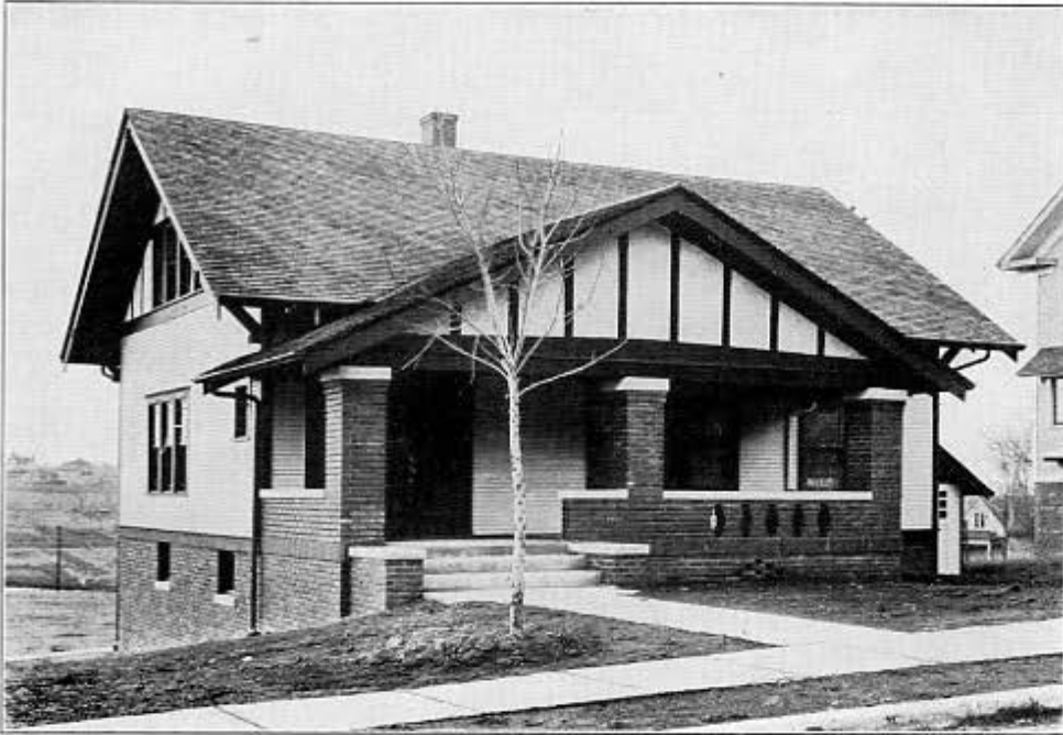
No. 250—This Handsome Bungalow is erected on Forty-first and Wakley Streets. Has four rooms on first floor and two rooms on second floor; is 38x30 feet in size. The massive brick pillars and gable of front porch with stucco panel gives the exterior a very massive effect.
