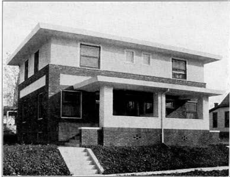
No. 228—This Duplex Brick and Stucco Combination Apartment is owned by H. D. Frankfurt, and located at Twenty-seventh and Poppleton Avenue. Each apartment has 5 rooms and sun-room, individual porches, upper part faced with pebble dash stucco. (L. E. Heifner, plumbing contractor. Glauber brass ware used. Milton Rogers furnished hardware. National Roofing Company furnished gravel roof. Burgess-Grandon furnished fixtures. Thew & Luhr furnished electrical wiring. Building faced with Hytex No. 207 press brick.)
