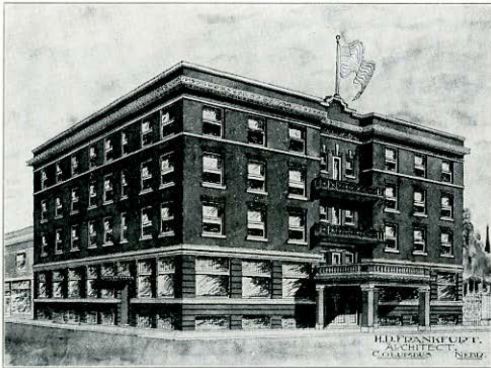
No. 204—Evans Hotel , built at Columbus, Nebraska, at a cost of $75,000.00, is four stories high, has 72 sleeping rooms, all fire-proof construction and modern in every respect. (American Gypsum block and plaster board used.)
