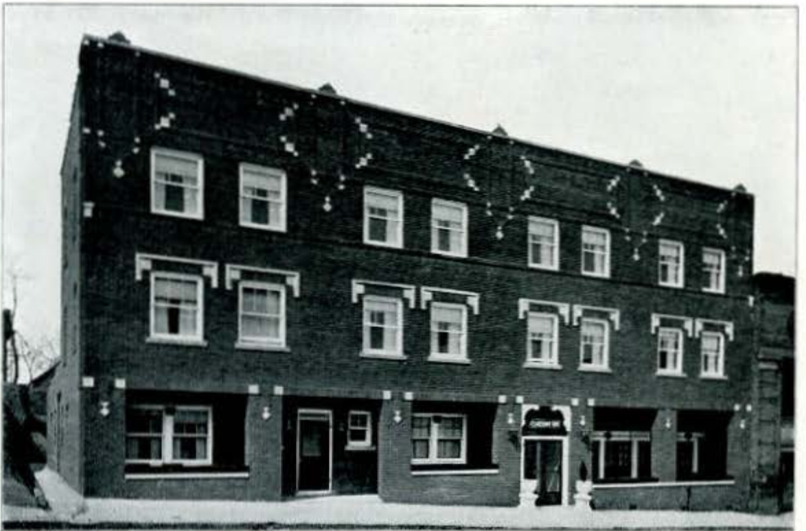
No. 210—Claremont Inn , located at Seventeenth and Jackson Streets. Owned by the Coad Real Estate Company. Has forty-eight sleeping rooms, four 2-room apartments, public dining room and kitchen. (Schollman Brothers, plumbing and heating. Monarch weather stripping used. Glauber brass ware used. Four Murphy In-A-Door beds used. Milton Rogers furnished refrigerators. Building faced with Sunderland's Brazil X press brick.)
