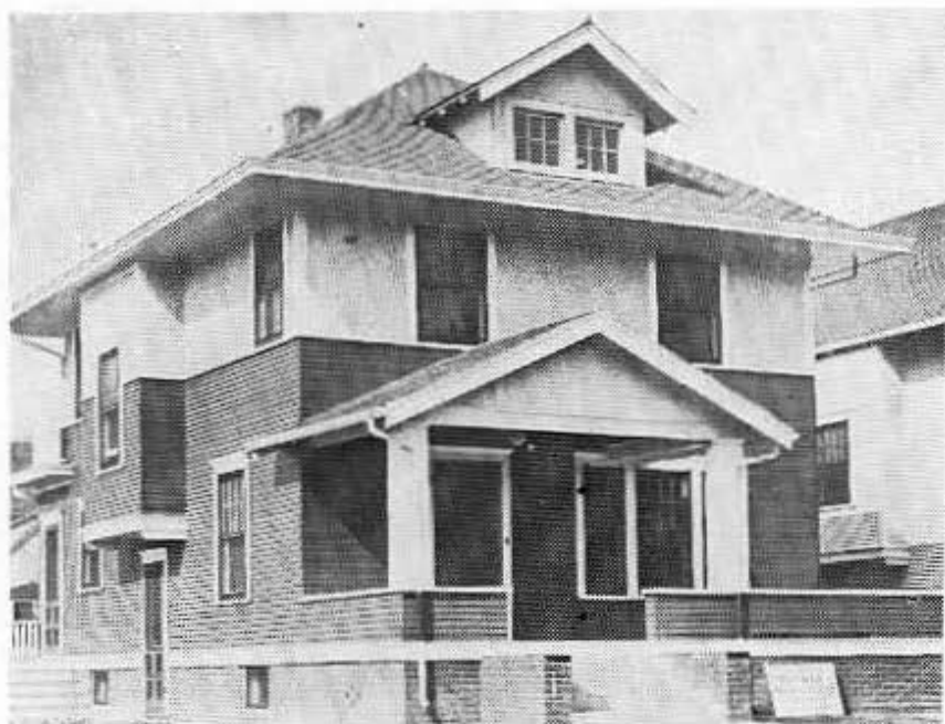
No. 245 —The Ground Plan of This House is 26x28. Has seven rooms, large attic, sleeping porch at rear, and large front porch. The upper part of house is stucco and is roofed with asbestos shingles, which makes a fire-proof construction.
