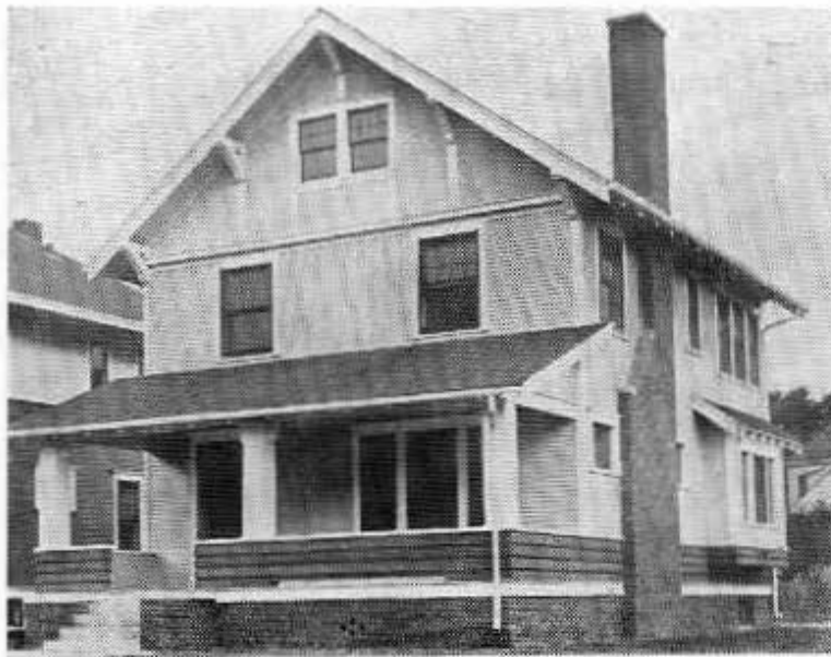
No. 242 —This Design gives a two-story bungalow effect, which is a very popular design. Heavy brackets support verge boards and bungalow siding is used around porch and base of building.
