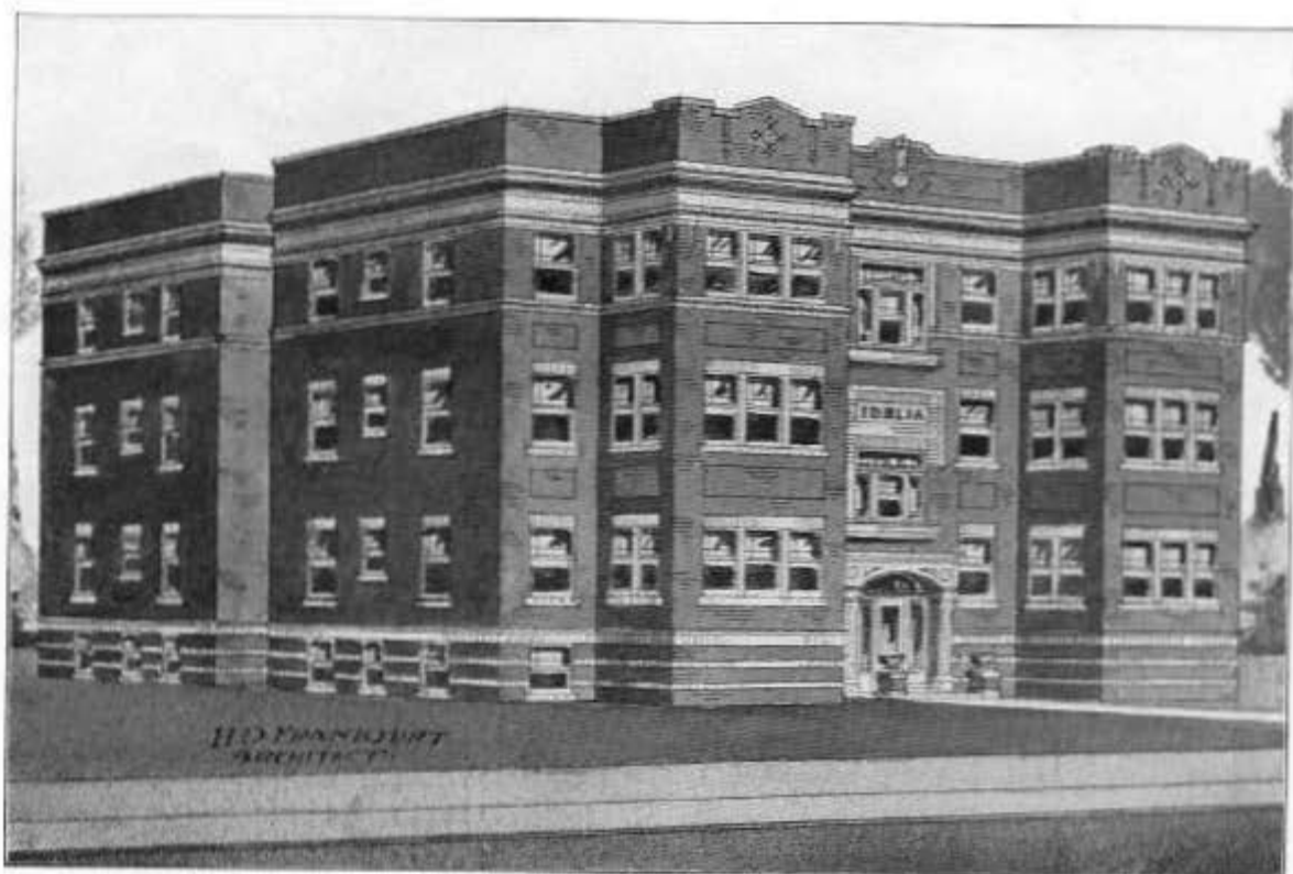
No. 214—Idalia Apartments , located on Thirty-third Street, between Dodge and Davenport Streets. Built and owned by Hastings & Heyden. Containing twelve 4-room apartments, each with large sun room. (Kerner incinerators used. L. E. Heifner, plumbing and heating. Milton Rogers, refrigerators. Monarch adjustable weather stripping. American Plaster Board lath used. Building faced with Sunderland's face brick. Glauber brass ware used.)
