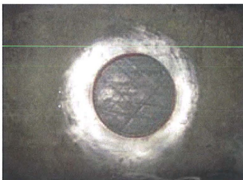
Figure 6. Test port of RF shelter seen from the inside with concrete slab and copper gasket.
