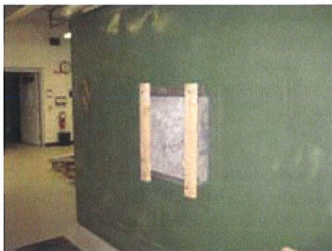
Figure 5. Concrete slab mounted on the outside wall of RF shelter.
