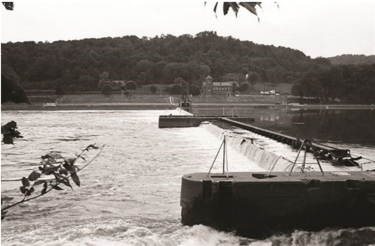
Figure 3. Ohio River wicket lock and dam number 18 at Reedsville, Ohio (USACE 3 n.d.).
