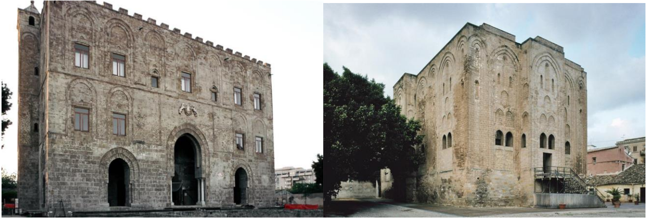
Fig. 8. Zisa pavilion, left. Cuba pavilion, right. Palermo. 1180.
