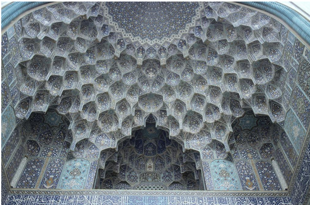
Fig. 9. Example of muqarnas. Shah Mosque, muqarnas. Ordered by Shah `Abbas I; finished under Shah Safi I. 1611-c. 1638.
