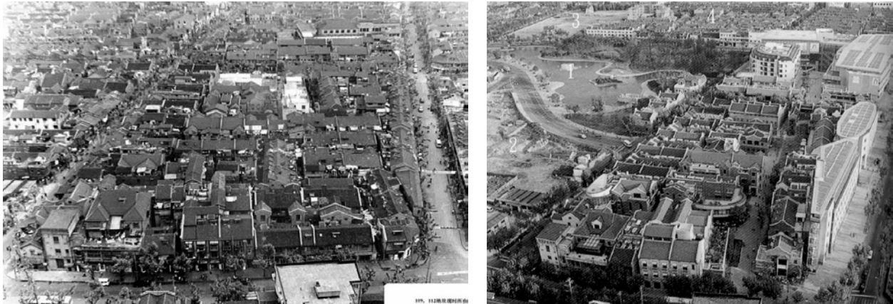
Fig. 3. The area before renovation (left); XTD after renovation (right)
