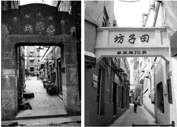
Fig. 4. Change of Shikumen houses in Linongs in TZF before (left) and after (right) renovation Source: Photo by the first author.
