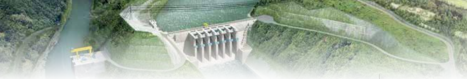
Photo Above: Pakistan's new Karot Hydropower Project
