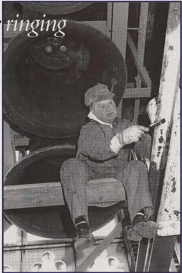
Restorers from Taylor Bellfounders of England worked on Trinity's carillon.
