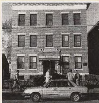
Vernon Street apartment building rehabilitated by SINA, late '80s.
