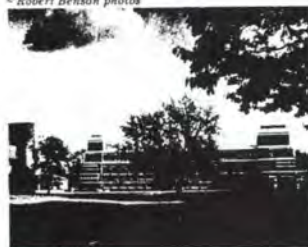
Along with the existing neo-Brutalist Jacobs Life Sciences Center (far left in top photo and overlay), Trinity's Mathematics, Computing and Engineering Center defines a
