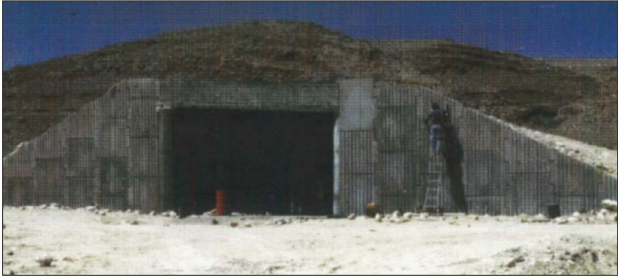
Figure 1. Protective Shelter constructed with Reinforced Soil
