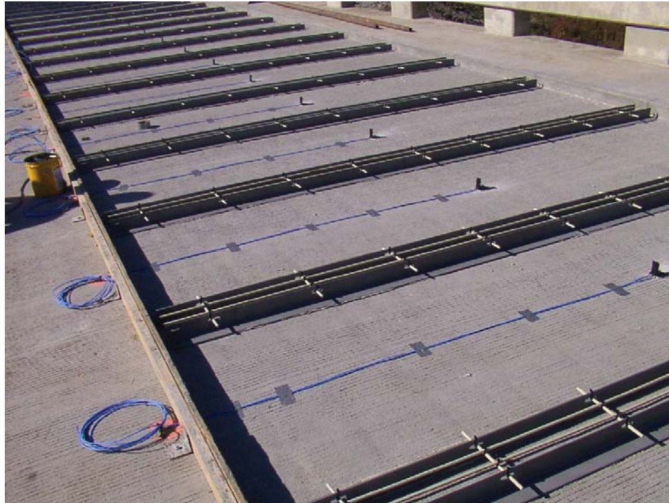
FIGURE 8 Electrode layout during construction.
