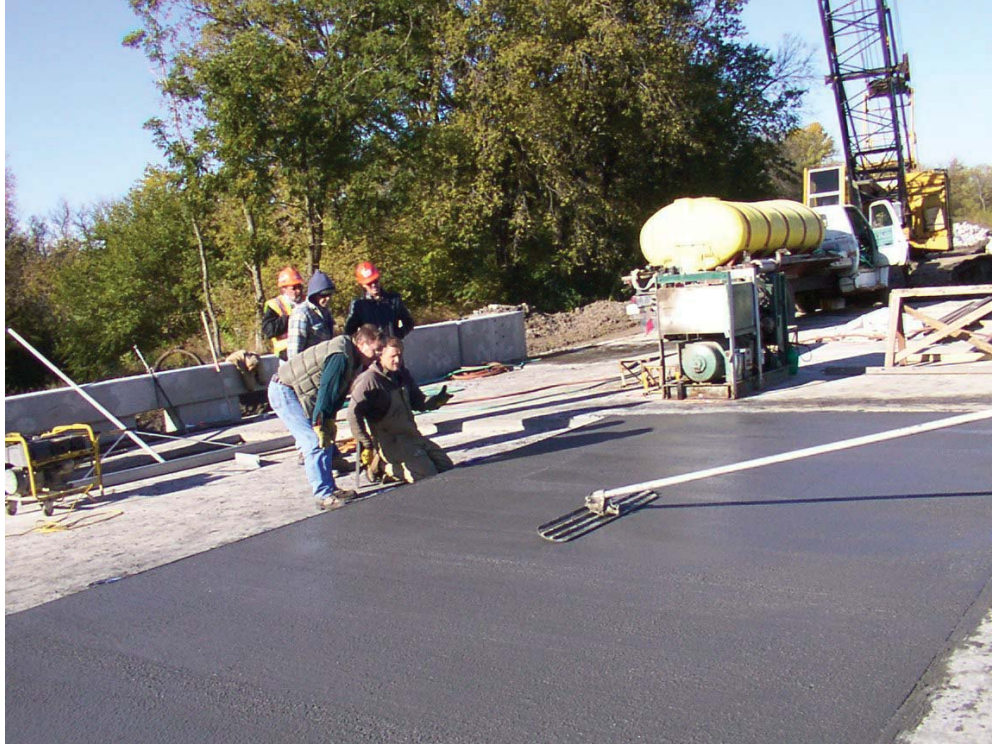
FIGURE 10 Finishing the conductive concrete inlay.
