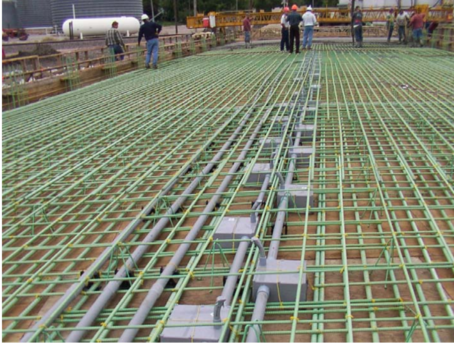
FIGURE 5 First conductive concrete overlay during construction at Roca, Nebraska.
