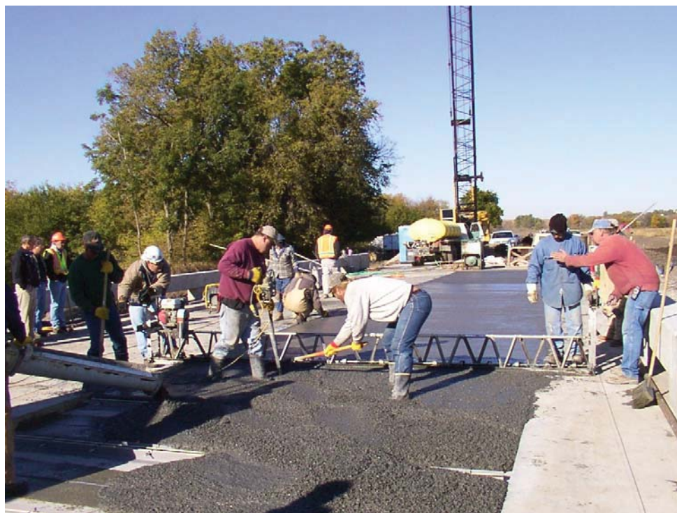
FIGURE 9 Casting the westbound lane with conductive concrete.
