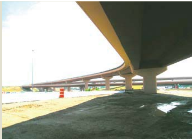
Figure 4. Summit Engineering Group designed a U-shaped, precast, post-tensioned concrete box-girder bridge for Interstate 270 that spans Interstate 25 just north of the U.S. Route 36 and Interstate 76 interchange in Denver, Colo. Courtesy of Gregg Reese, Summit Engineering.
