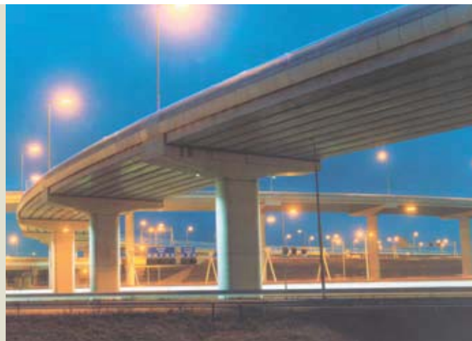
Figure 1. A curved, pretensioned concrete box-girder bridge in Rotterdam, Netherlands, is a prime example of standard practice for bridges in the Netherlands for more than a decade. Courtesy of Spanbeton.
