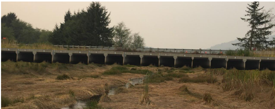
Figure 14. Multiple culverts along Hwy. 101
