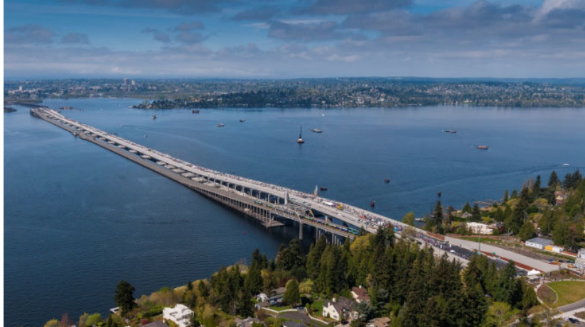
Figure 11. Evergreen Point Floating Bridge (WSDOT, 2018)
