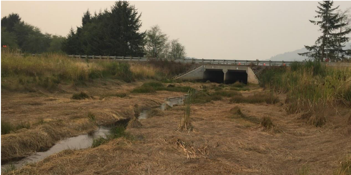
Figure 5. Fraser Creek Culvert (Ellingson, 2018)
