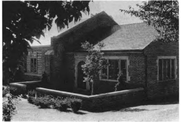
Figure III-10 Hallden Engineering Laboratory
