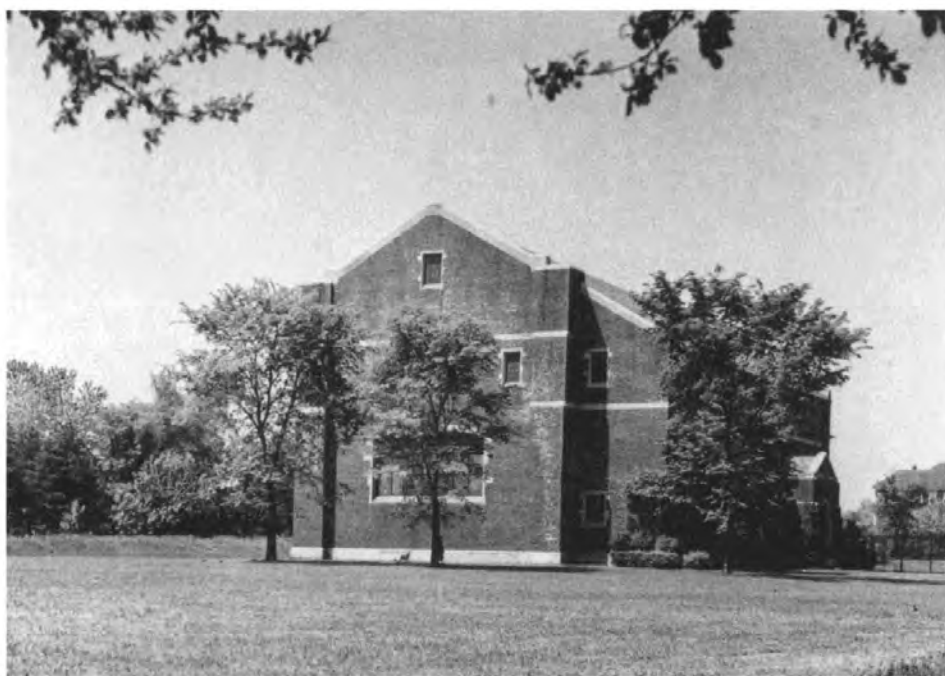
Figure II-9 Trowbridge Pool and Squash Courts
