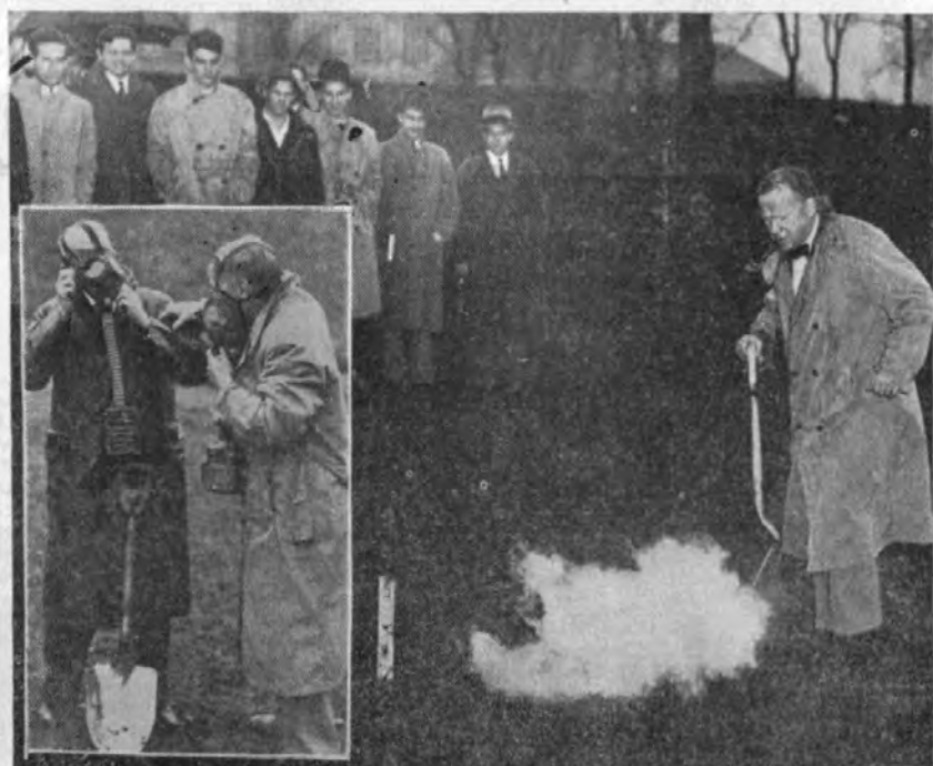
Prepared chemicals caused smoke to issue from the ground as President Ogilby turned over the first spadeful for the new Chemistry Laboratory. Insert shows Dean Hood and the President donning gas masks preparatory to the further conquest of "Chemistry Bluff". (Courtesy of "Hartford Times")
