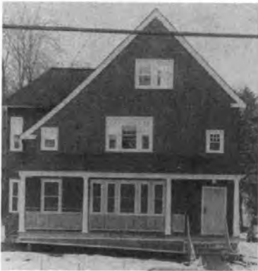
Fig. VII-9 Umoja House shortly after its relocation to 74 Vernon Street
