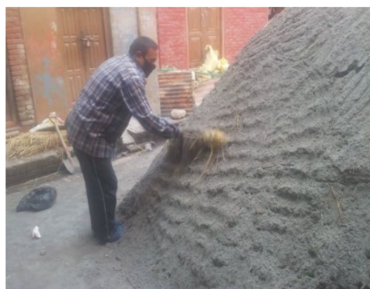
Figure 8: Stabilizing Ash Walls
