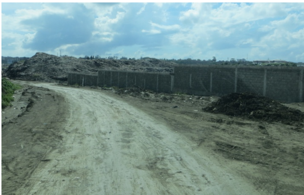
E5: Construction right at the edge of Kibarani dumpsite
