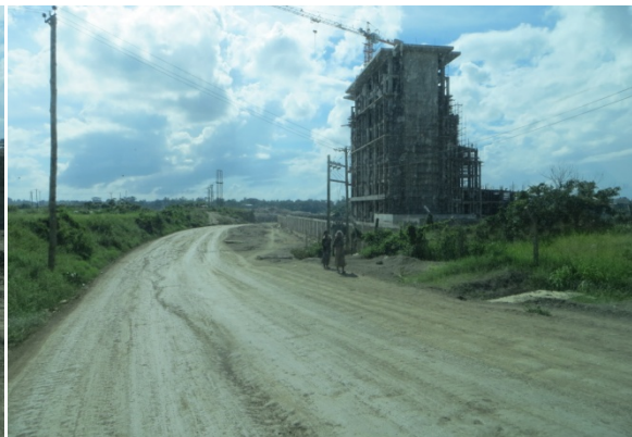
E6: Office constructed on cleared Kibarani site
