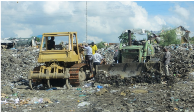
E3: Bulldozers leveling the trash
