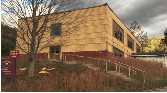
This Diana Elementary School building was in use up until 2002.
