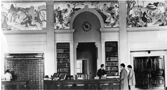
1940 view of Morrow Library reading room showing original configuration of the Fors Murals.
