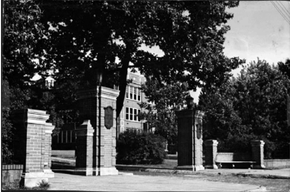
1940 view of Marshall's 4th Avenue and 16th Street (now Hal Greer Blvd) entrance gate before the plaques were removed.
