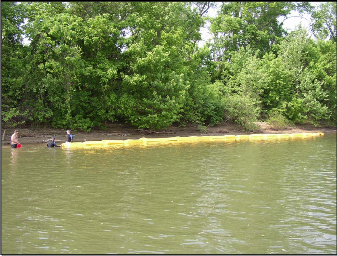
Figure 15. Floating turbidity exclusion fence setup along the Kanawha River, West Virginia
