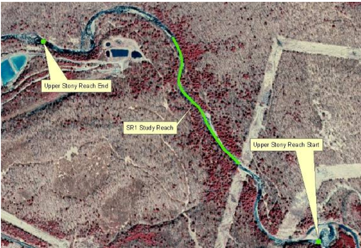
Figure 3.2. Upper Stony River Reach Aerial Photo
