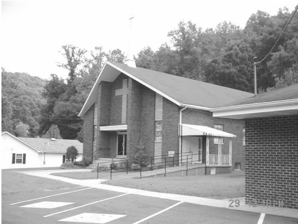
Image 1 - View of the Outside of the Church, Author's Photo
