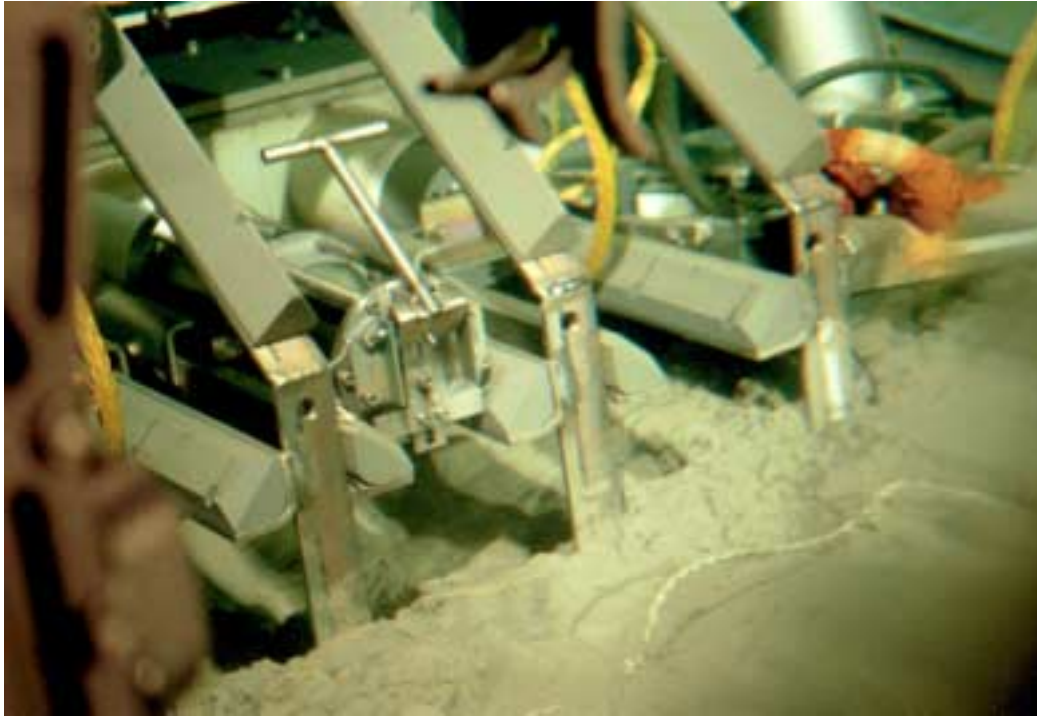
Figure 7. The HUGO Junction Box on Loihi. A hydrophone is connected in one of the instrument bays. The front of the package is buried about 30 cm in the mud.
