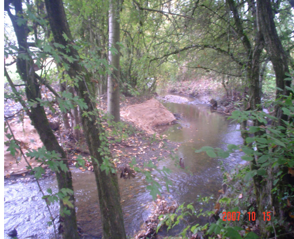
Figure 5. Usual flow conditions illustrating erosion and mitigation along the channel.
