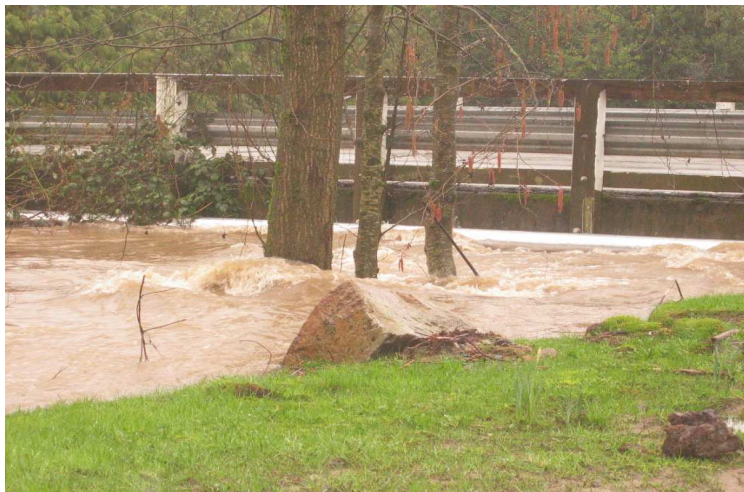
Figure 8. Debris damaged gas line that crosses the channel at the Wright Street bridge in Clayburn Village.
