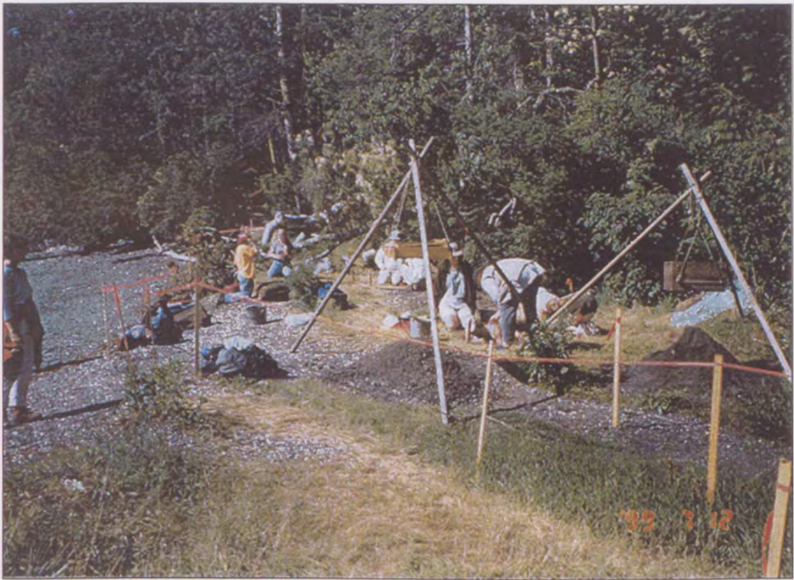
Figure 6. Photo of excavation at SK-144. Lottie Bay is to the left of the photo.
