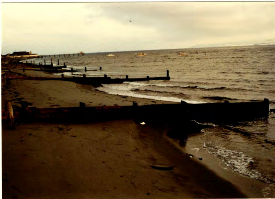
FIGURES 8a and 8b. Photographs illustrating the effect of an object interrupting net shore-drift. Photo 8a shows an individual groin in the groin field depicted in photo 8b. These photographs were taken looking north and west respectively in Drift Cell 3-1.
