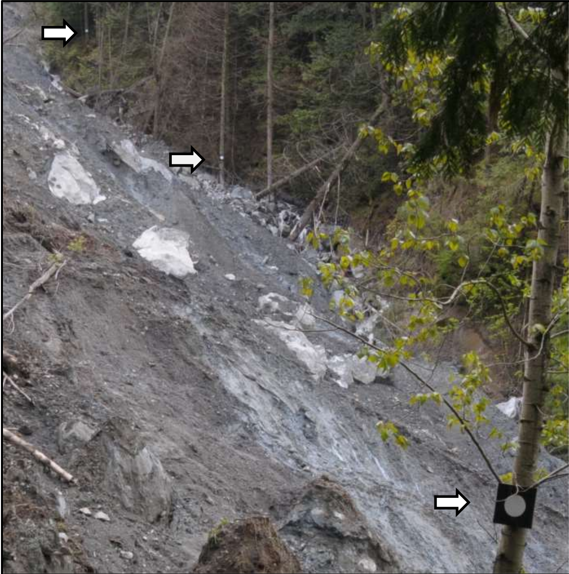
Figure 8 - Photo of the north side of the landslide (May, 2010), showing the network of three artificial targets mounted on stable trees. One target is in the lower-right foreground and the other two are in the upper-left background. The forest and exposed bedrock in the background served as the stable terrain for this study.
