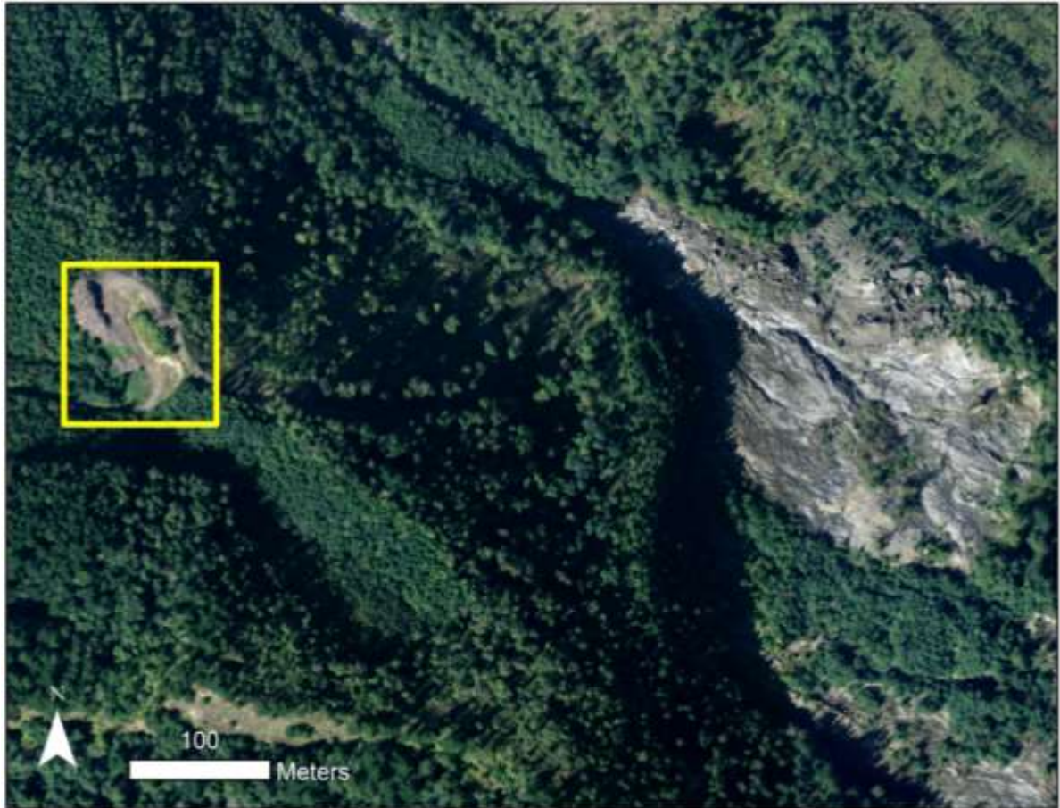
Figure 3 - Aerial view of the toe of the landslide. A nearby logging road, framed in yellow, was one of two road surfaces used to check for discrepancies between the 2006 and 2011 airborne LiDAR datasets (Road B is pictured above).
