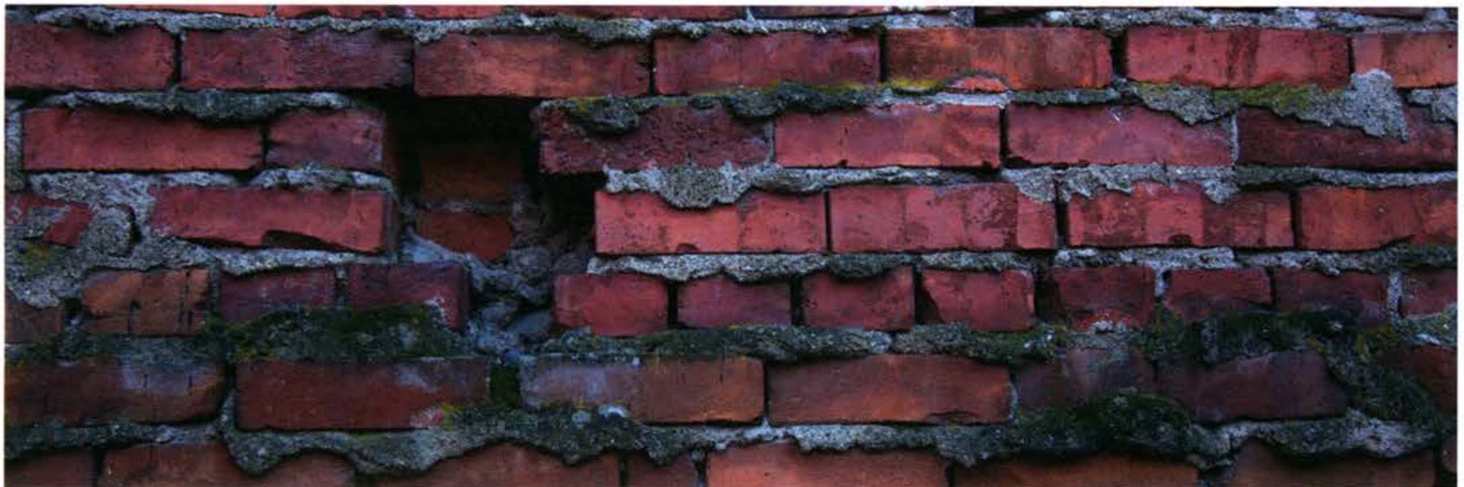
BELOW: Burnt clay bricks are the most common and among the most risky building materials for earthquake safety, Tinner said.
