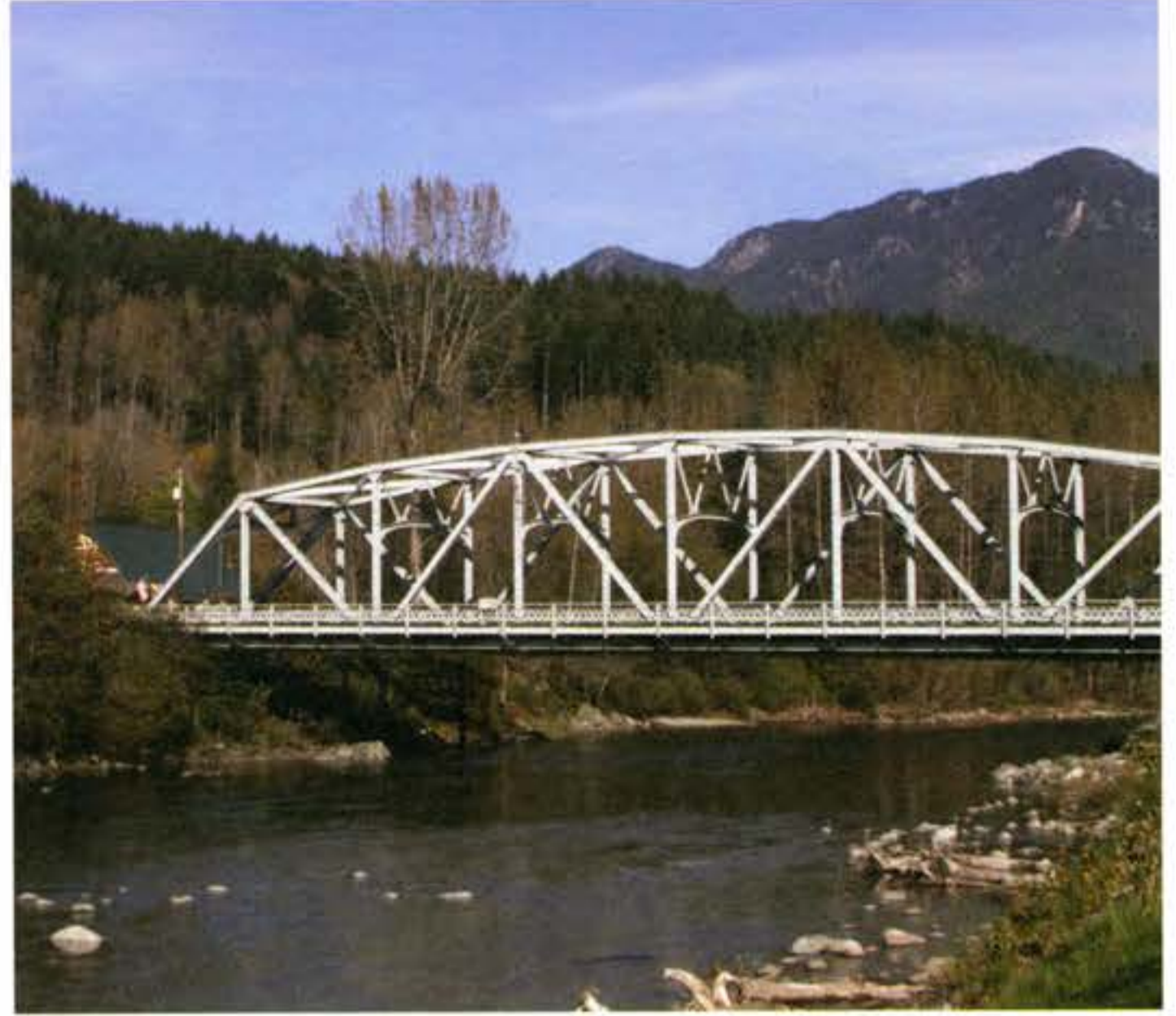
▲ The Skykomish River, with the bridge that crosses it into the town of Skykomish, Wash. Bunker C fuel was discovered to be seeping into the salmon habitat of the Skykomish River in 1996. The oil had been pooling underneath the buildings of the town, accumulating in the soil.
